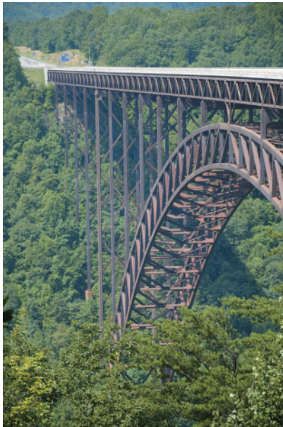
The New River Gorge Bridge in West Virginia is the longest arch bridge in the United States.
